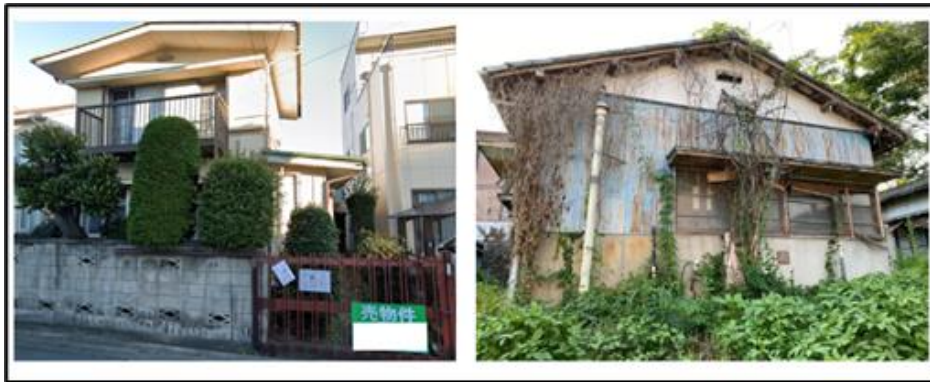
Figure 7. Example of the exterior of a building with a high probability of vacant house that falls under FP
